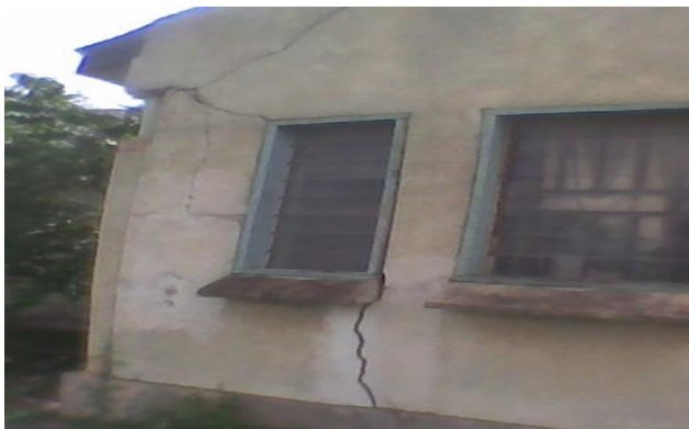
Fig. 1. Cracks on building founded on shale deposits located at the College of Engineering, University of Agriculture, Makurdi, Benue State, Nigeria (Iorliam et al. 2012b).
